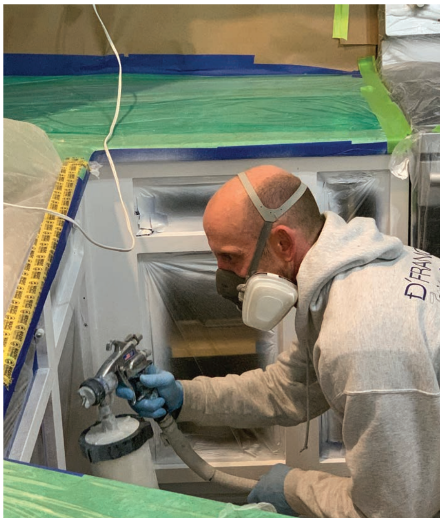
Helmrich topcoats a kitchen cabinet.
